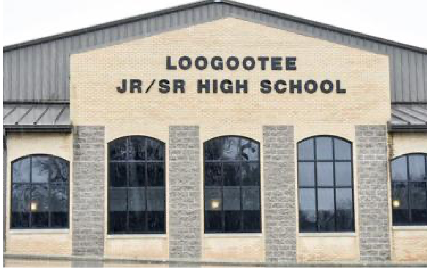
Photo of Loogootee Junior/Senior High School in Loogootee, Ind. (Photo via Washington Times-Herald)
